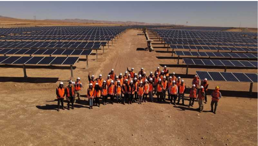
Figure 45: Solar plant for BHP
